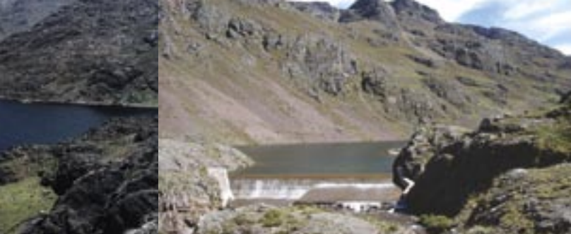
Aliviadero Chungará / Spillway at Chungara
