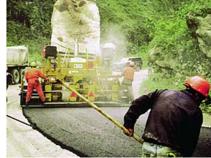
Carretera Tabinapampa-Tunquini (1998) Tabinapampa-Tunquini highway (1998).
