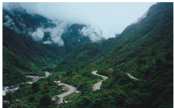
Carretera Tabinapampa - Tunquini: Sector Chacaneque Tabinapampa Tunquini Road at Chacaneque village
