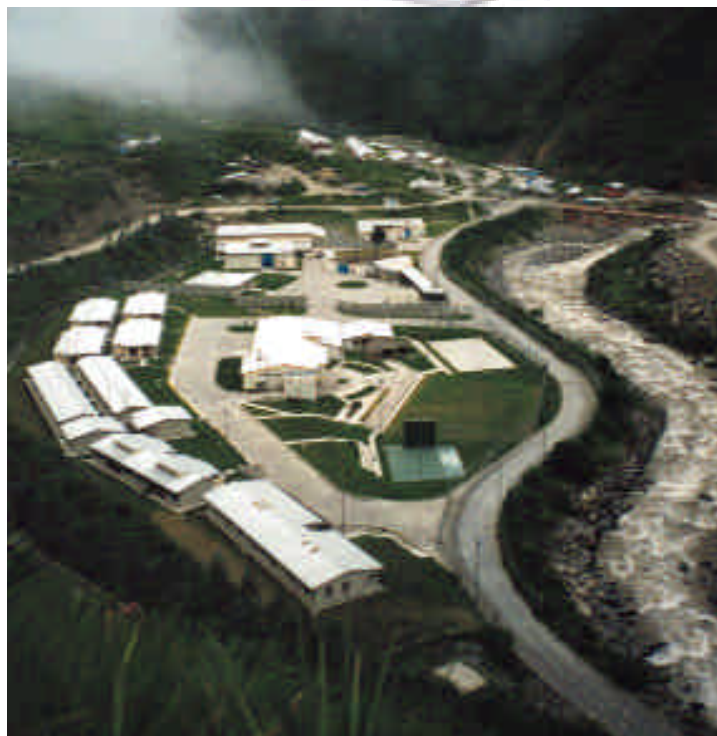
Villa de Residentes, Sede Administrativa y Obras de Cabecera de la C.H. San Gabán II Residents Village, Administrative Offices and Headworks of The San Gaban II Power Station
