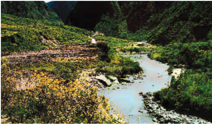
Chuani - Zona donde se construyeron las Obras de Cabecera Chuani - Site where Headworks were built.
